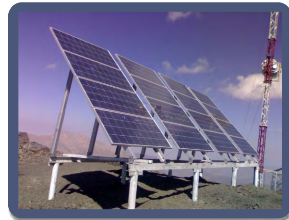
■ SAF CFM powered by solar panels
